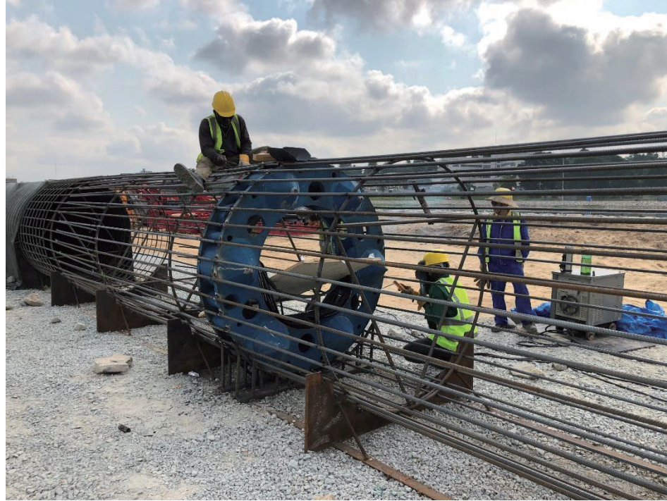
b) Welding with steel cage
