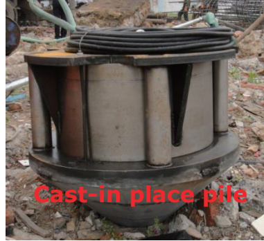
Cast-in place pile with Single link
