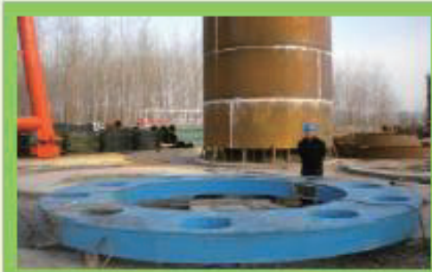
Annular load cell for caisson
