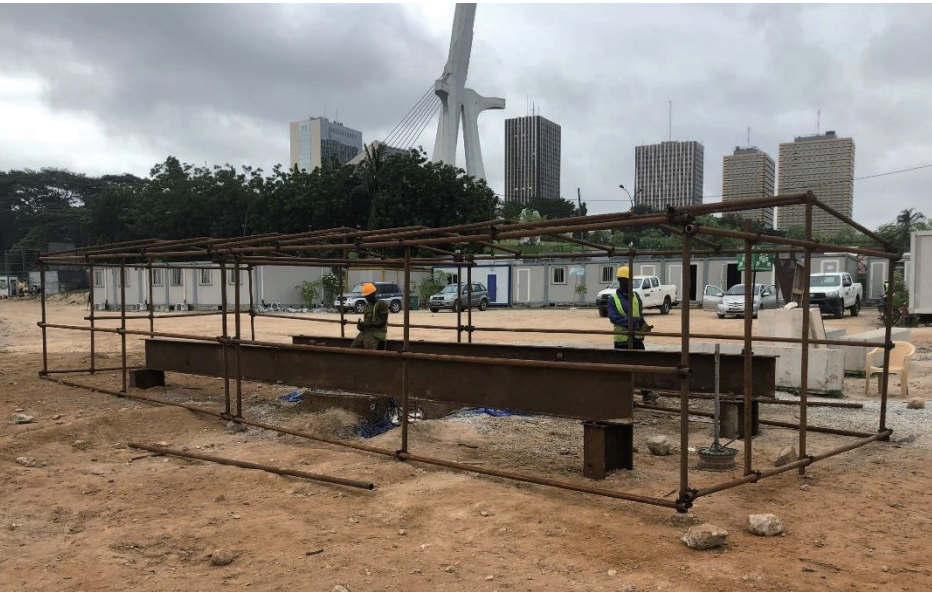
a) Erection of reference beams
